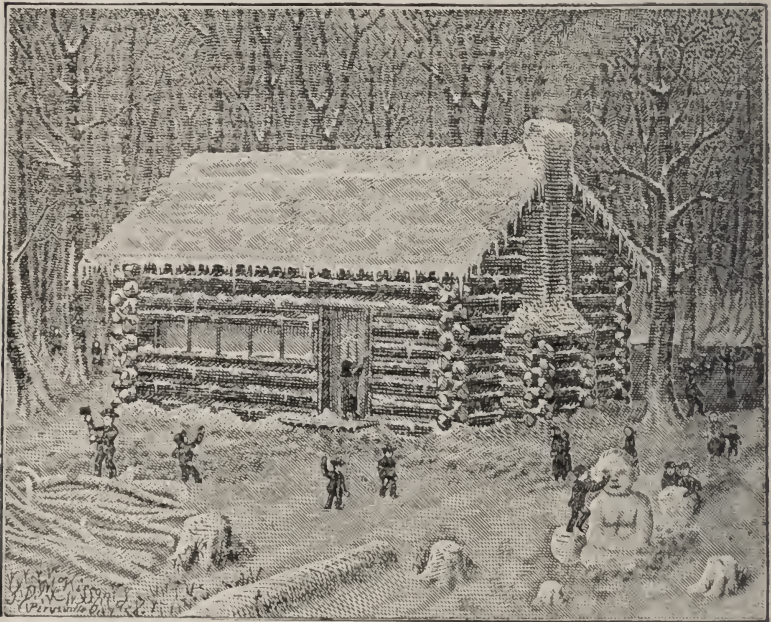
FIG. 1. LOG CABIN SCHOOL HOUSE.
